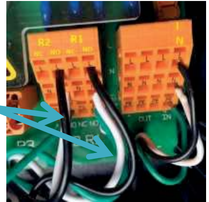
Figure 23 Terminating R1 & R2
